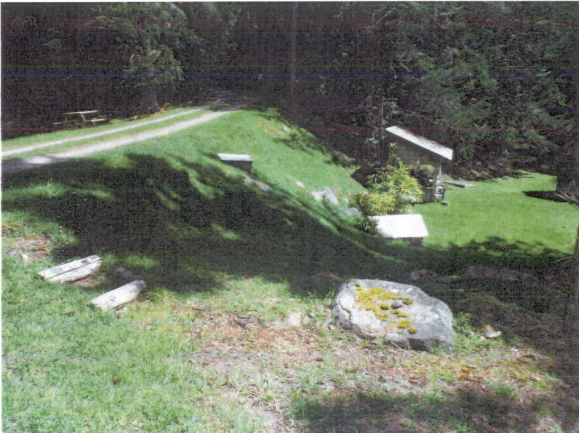
Gardom Pond Dam – Downstream face of dam.
