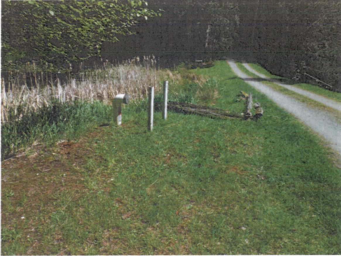
Gardom Pond Dam – Remove vegetation on upstream face of dam.
