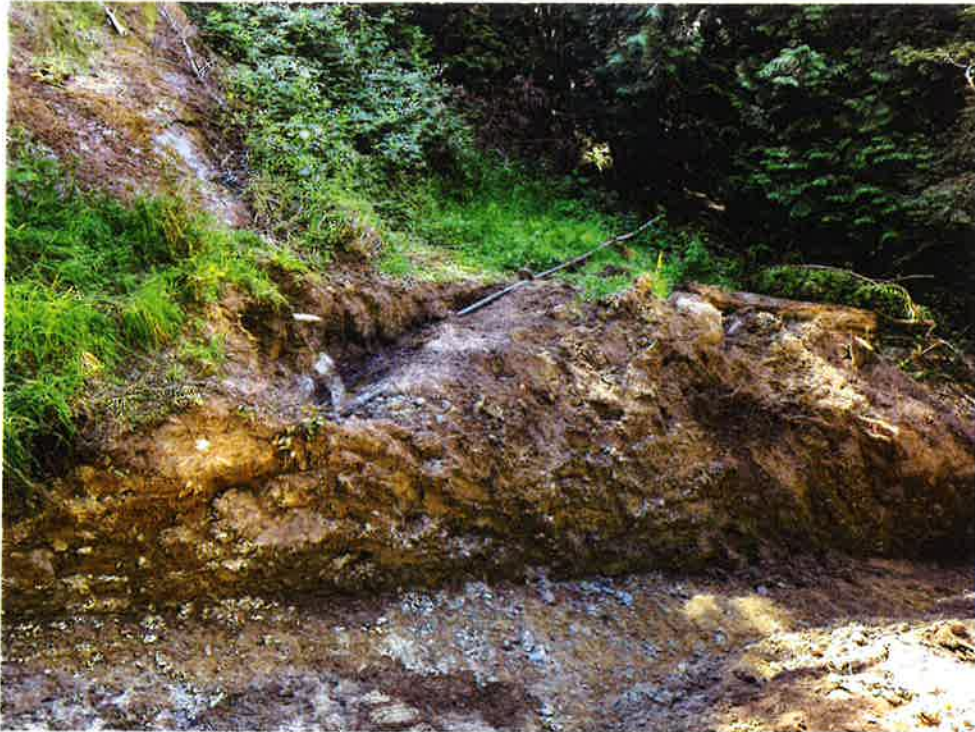
RPID diversion ditch. Mostly completed. 2" line (right) and 4" line (left by shovel) exposed.
