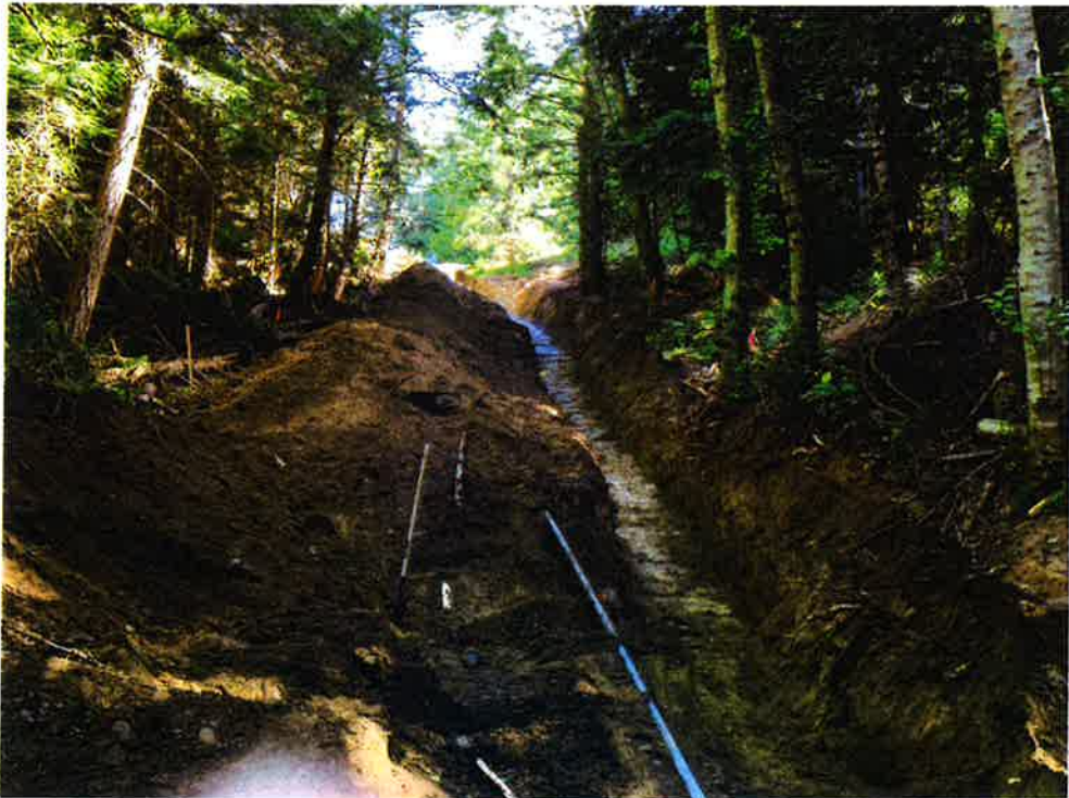
RPID diversion ditch. Mostly completed. 2" line (right) and 4" line (left by shovel) exposed.
