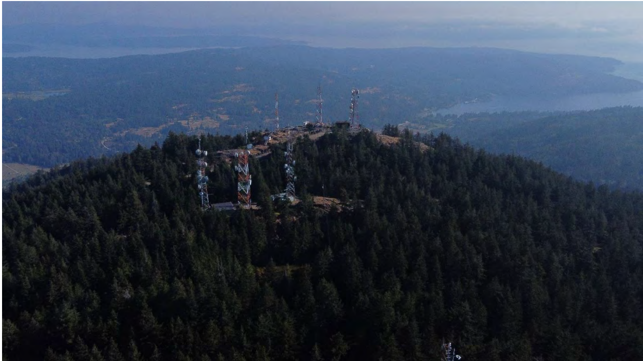
Photo 5. Communications infrastructure on Mount Bruce in SSI.
