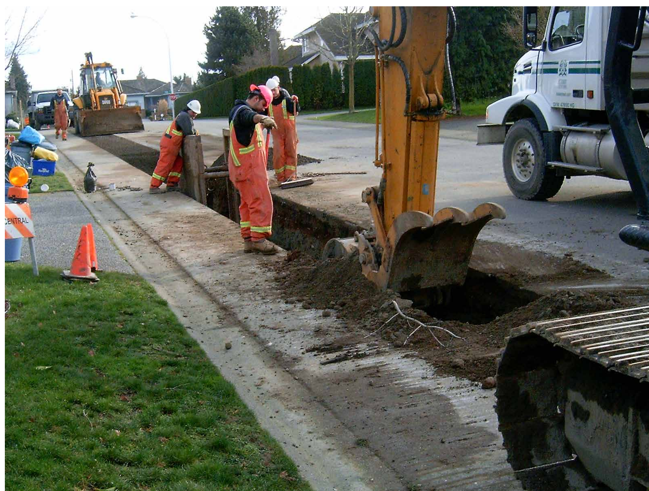
Conveyance pipe installation
