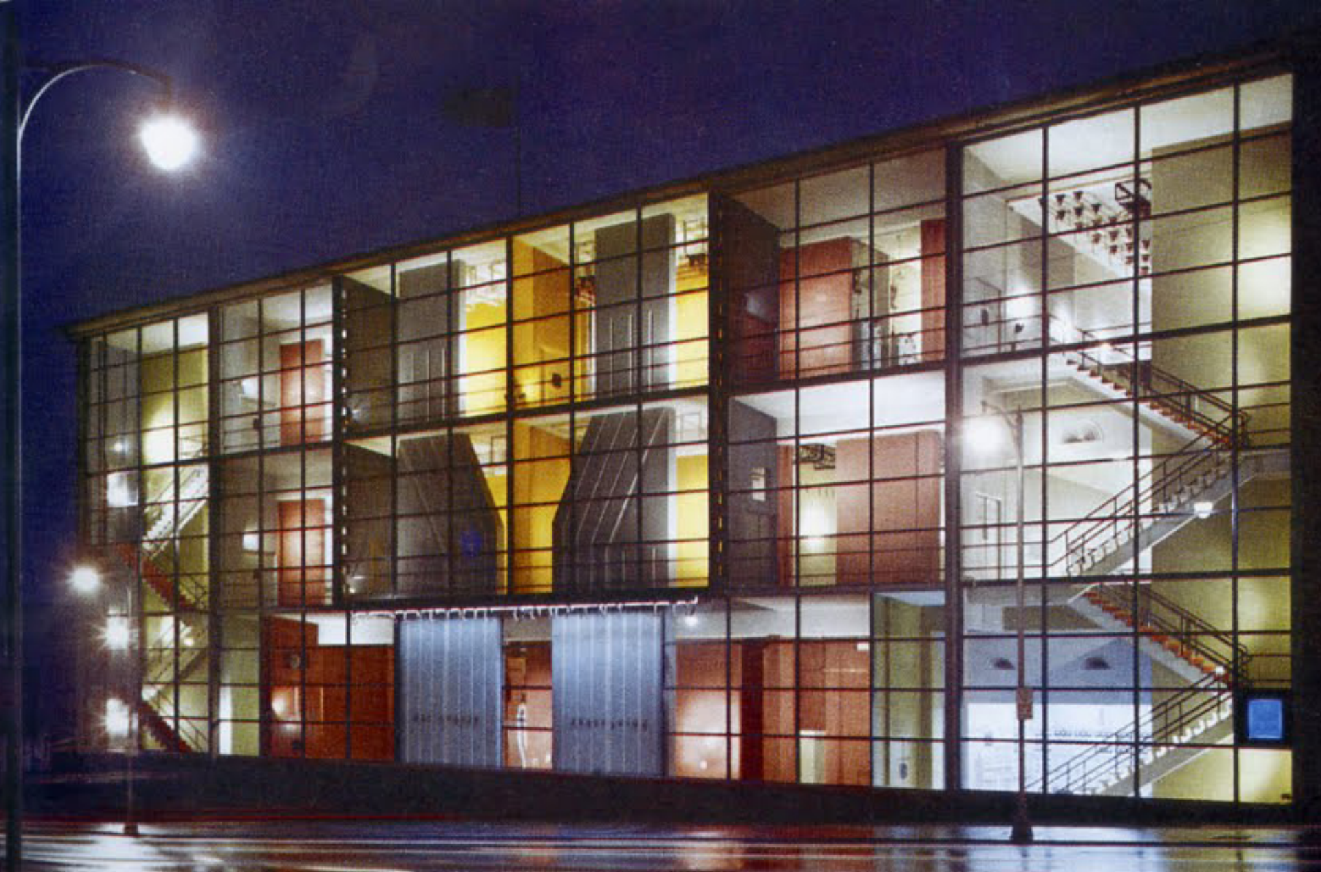
Dal Grauer Substation, Burrard Street (Architect: Thompson, Berwick and Pratt) Vancouver, BC
