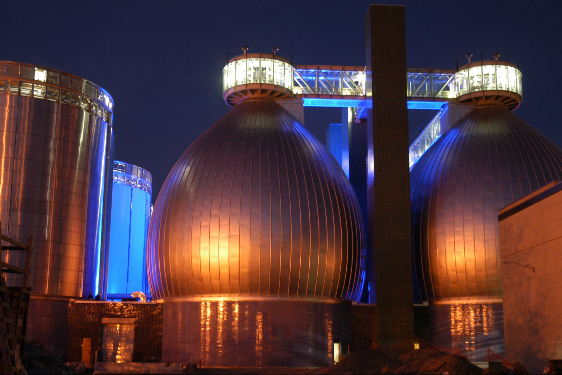
Newton Creek Wastewater Treatment Plant (Architect: ENNEAD) Brooklyn, NY
