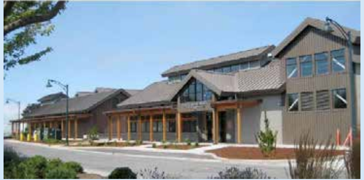
Pictured above is a wastewater treatment facility located in Blaine, Washington.
