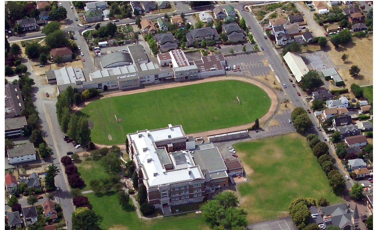
Aerial View (prior to demolition)
