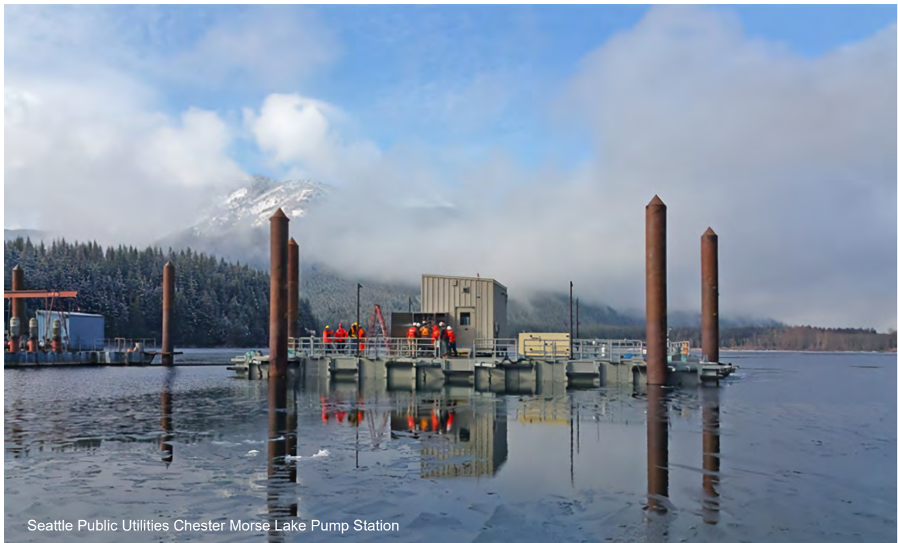
Figure 4.15: Floating Pump Station
