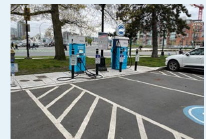
Example of on-street perpendicular parking with EV charging (Store Street, Downtown Victoria).
